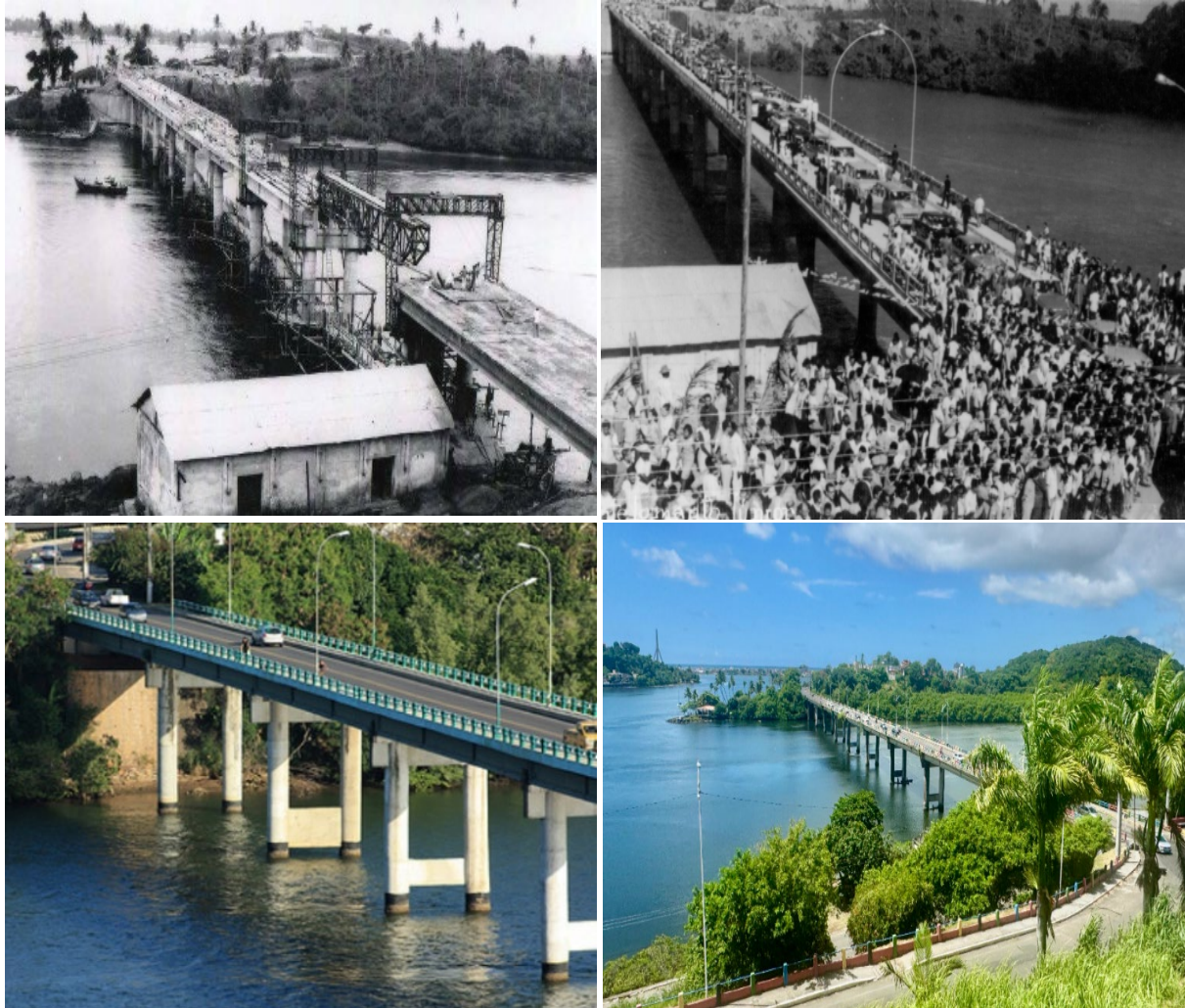
Figure 6. Inauguration of the Lomanto Jr. Bridge on August 15, 1966, and recent images from 2000 and 2025.
